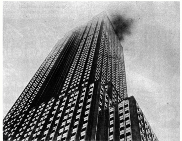
162 fire alarms in six minutes for the Empire State Building
