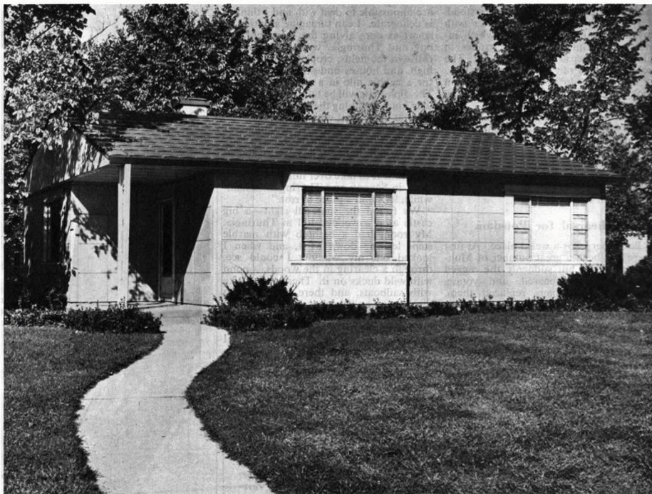
Lustron officials claim that bottlenecks in mass-producing the home are just about eliminated. But the problem of distributing the prefabricated units still remains
